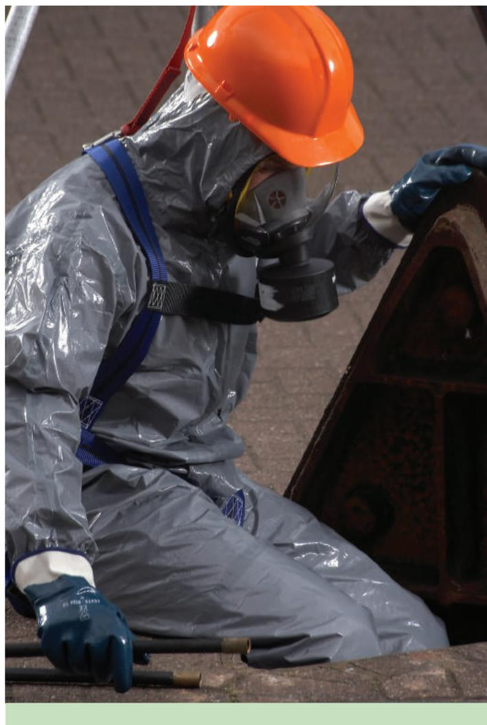
Superior multi-layer barrier films laminated to spunbond PP substrate - 170gsm.
